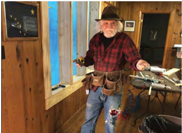
Tony Goggans replacing windows.
