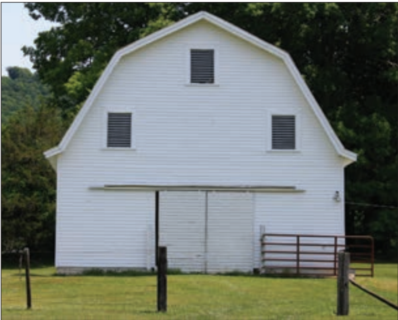
The original main barn was destroyed by fire and replaced in the 1940s.
