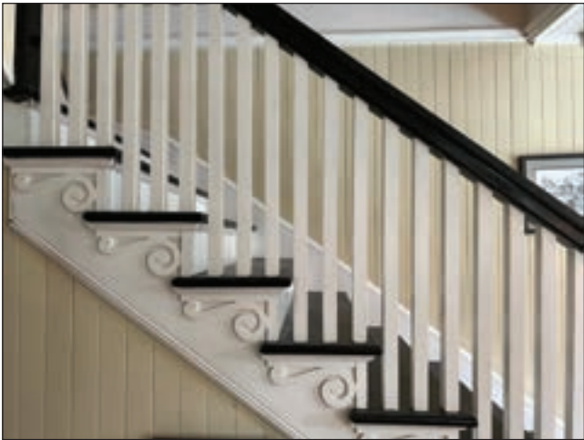
The grand staircase features original architectural details.
