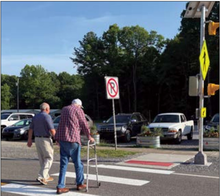
A new pedestrian crosswalk has been installed in front of the Mentone Market. With the push of a button, solar-powered flashing lights alert drivers to stop. Pictured are Mayor Hammond and Gerald Bailey.
