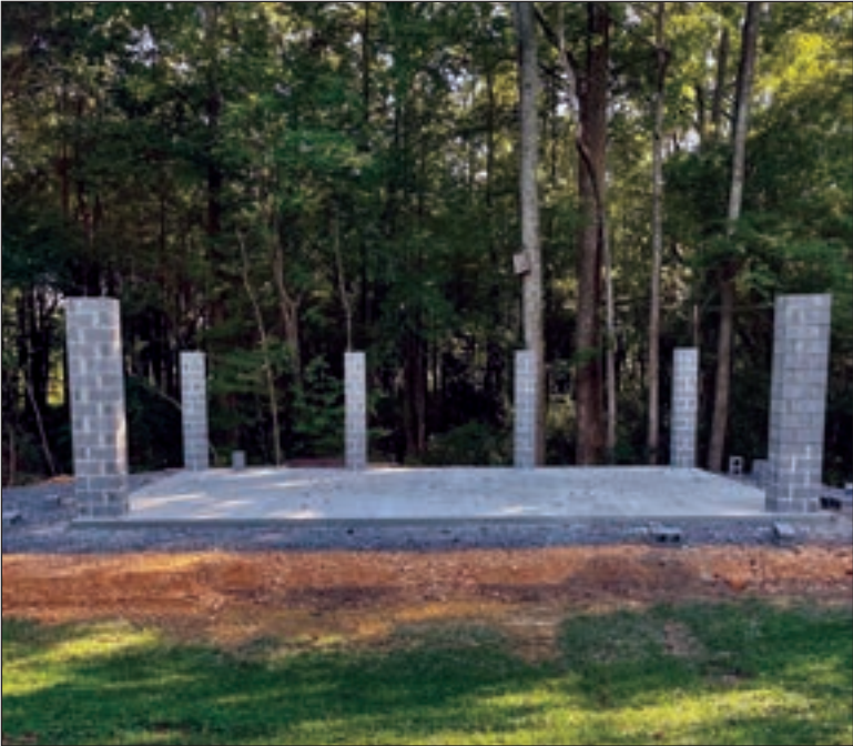
A work in progress: The stage is getting ready for a roof 8/30/22
