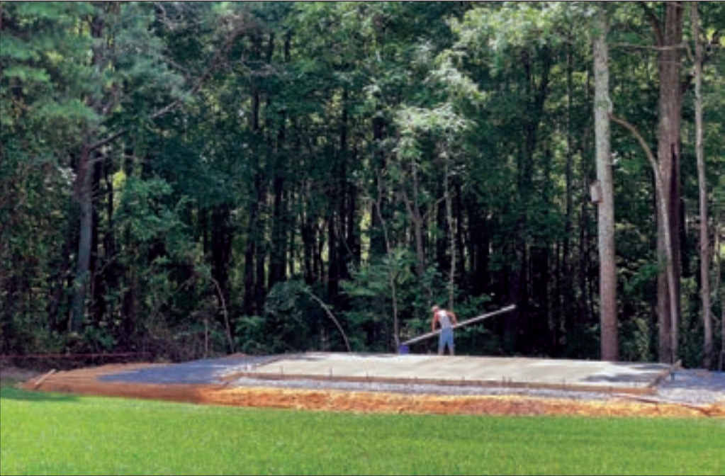
The foundation has been laid 8/4/22
