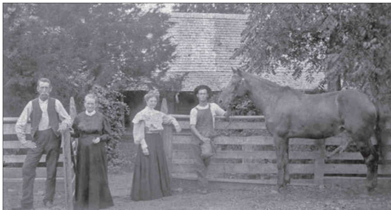
The original two-room cabin, built before the Civil War on property originally homesteaded by Billy and Nan Jones. Until the Cottage was built in 1921, only this house and a hilltop barn stood on the property. This turn-of-the-century picture features (L to R): William Taylor Jones, Emma Tabitha Jones, Nettie Jones Green, and Leonard Matheny.
