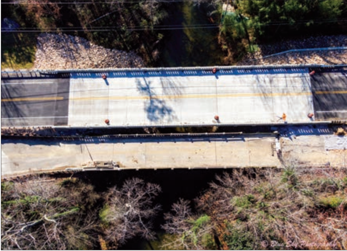
Charlie Stone of Blue Sky Photography has been flying his drone to capture aerial views of the bridge as a way of documenting the construction. Above is his most recent image, taken on November 20, 2020.
