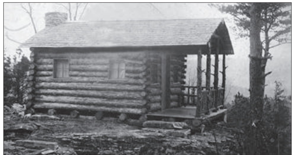
Colonel Howard's cabin. Note the unique foundation, necessary since the cabin was built on stone. The chimney remains standing. Photo credit: AP, courtesy of Joel Leonard
