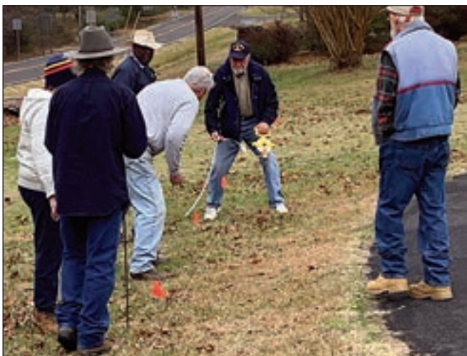
The Pathway to Community fence team marks the placement of the fence posts along the walking trail.
