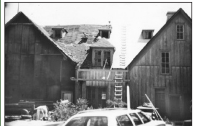
Roof repair in 1981 - Photo By Ray Padgett
