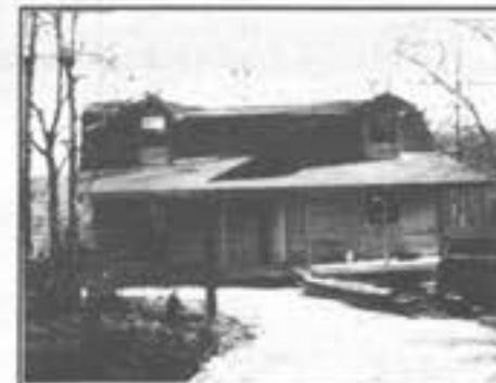
(2) NEW LAKE HOUSE - Under construction is this 3 bedroom, 2 baths, cedar exterior fireplace, located on Lake Labuaga. Great for vacation or permanent residence. Priced to sell at $75,000.
