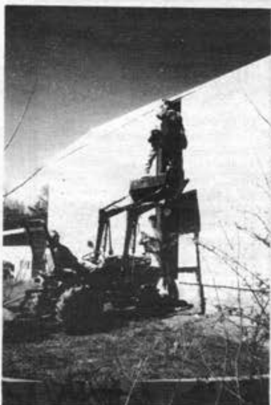
Milton Chambers operating the equipment, Eric Kirby drilling holes, and Rusty Chambers standing on ground
