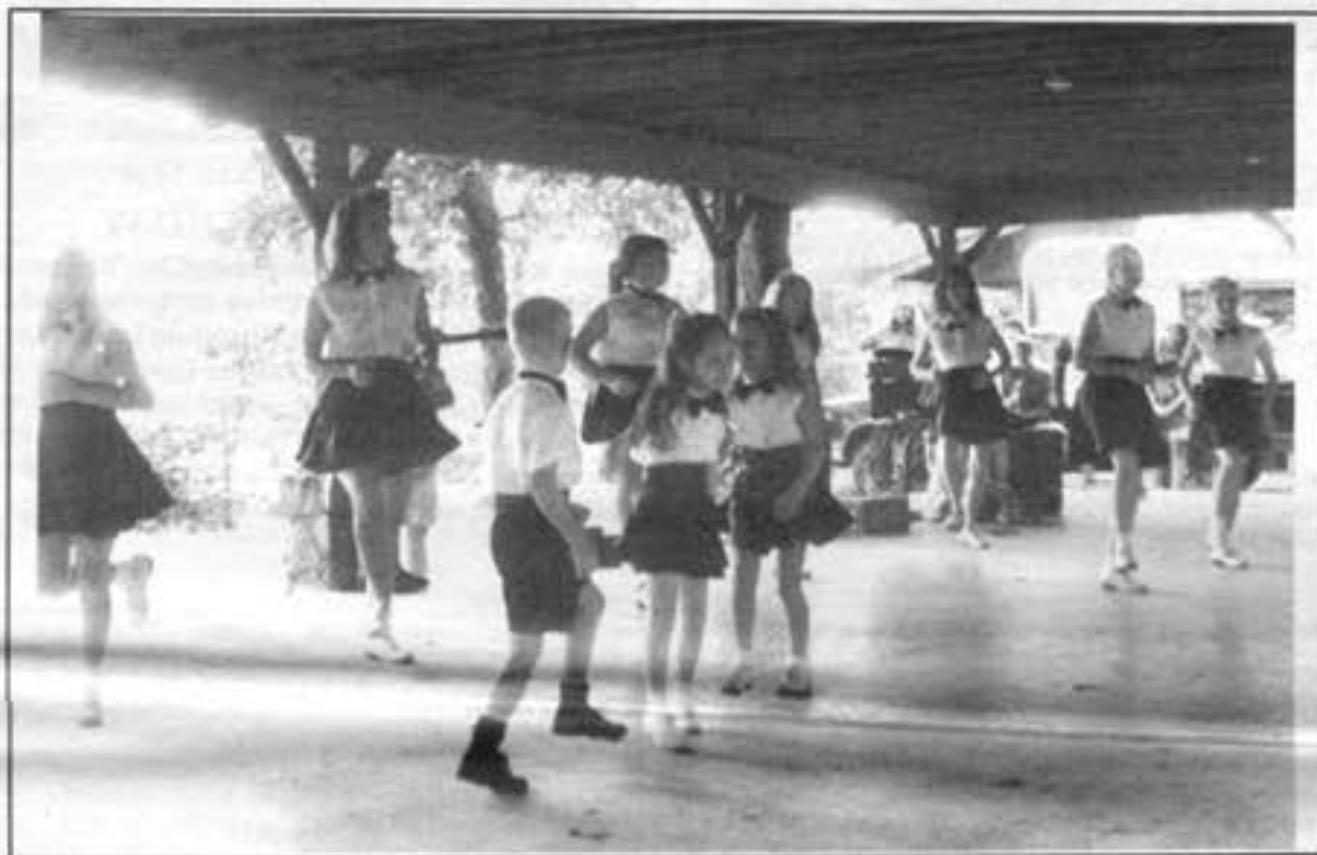
Clogging atop Lookout Mountain
