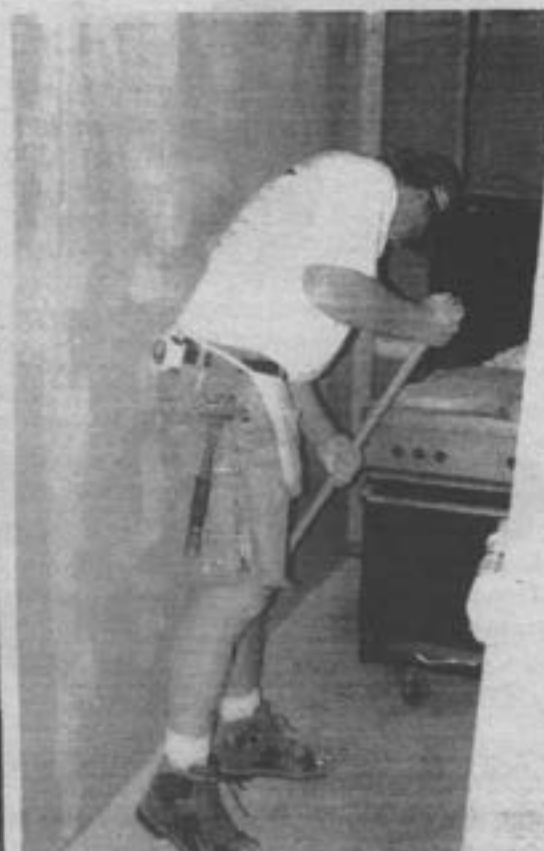
Pastor Rick Haworth sanding drywall
