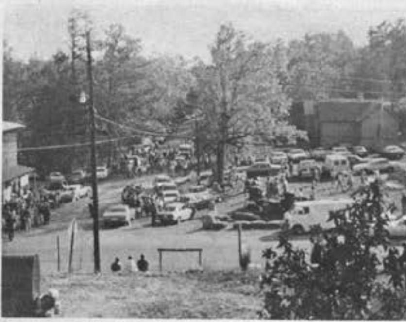
An over-all view from the porch of the Mentone Springs Hotel...
