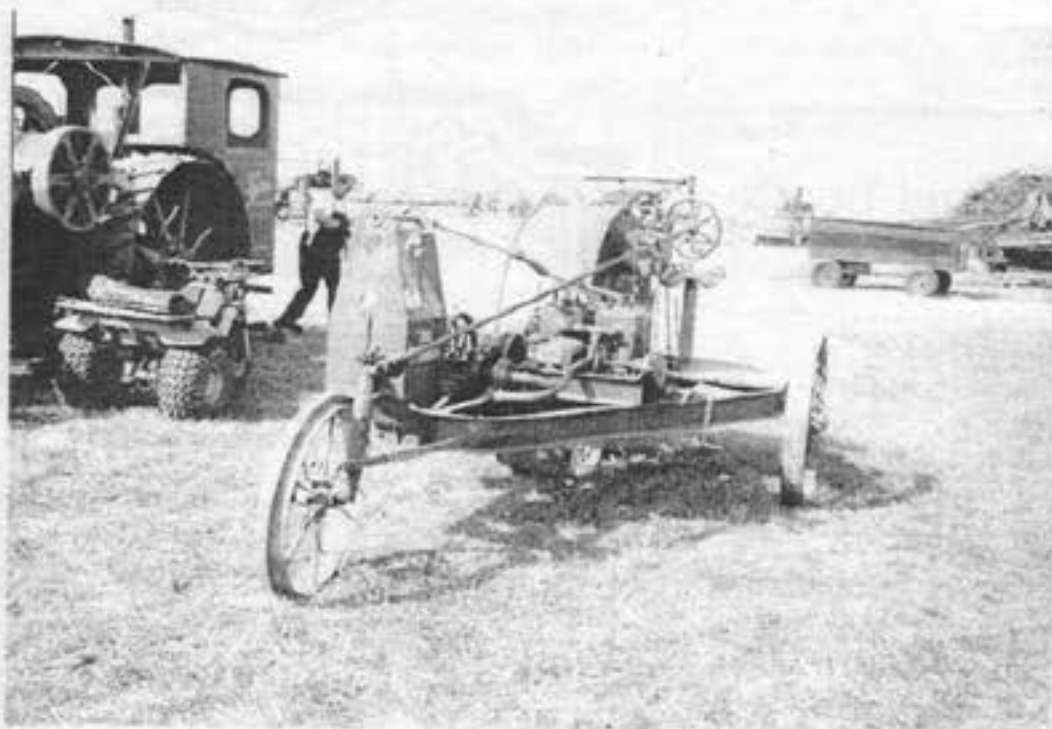
Early 1890s (radiator is to the side) One wheel pulls and one holds the tractor up.
