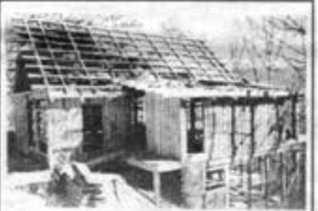
HWY 117 - MENTONE, Ala. - Mountain River Estates-3.48 +/- acres with road frontage, and 400+ ft. of river frontage overlooking the middle fork of Little River. Approx. 2300 sq. ft. cabin style home under construction. Beautiful natural foliage, rhododendron, and mt. laurel provide the quiet setting and privacy of this mountain home. $149,500. (No. A-50)
