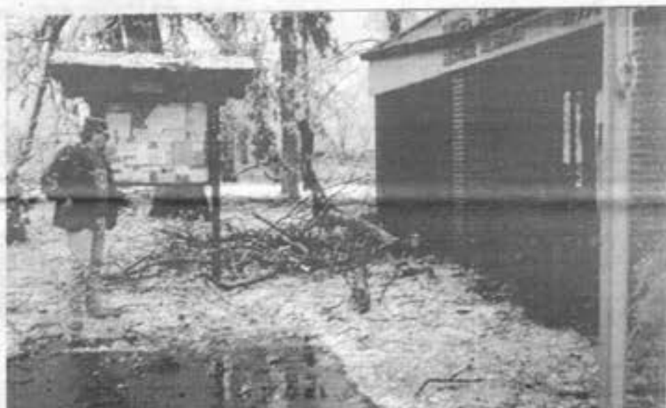
Benny Goss, Mentone Postmaster, surveying the damage to the front of the Post Office building. Much of the debris was later removed by Creative Tree Service out of Tennessee, hired by the Alabama Department of Transportation to clear Hwy 117 after the ice storm. They were using a chipper that "ate whole trees." Many downed trees and branches lined the highway all the way to the Georgia line.
