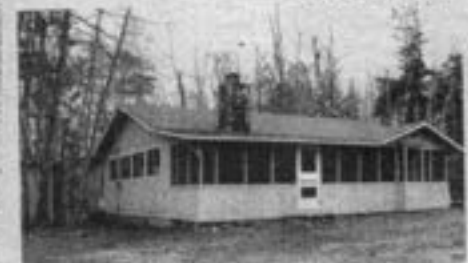
(4) MENTONE COTTAGE , all new plumbing. Stone fireplace. Remodeled with new flooring throughout. Sits on 3 lots. 3 bdrm 1 bath. Screened porch & fenced. $73,500.
