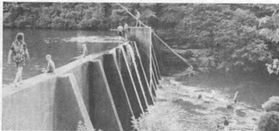
MILLER DAM though originally built as a hydro-electric project, now creates a swimming area for Little River at the Falls. Swimmers like the area behind the falls. Other visitors wade in the pools below.
