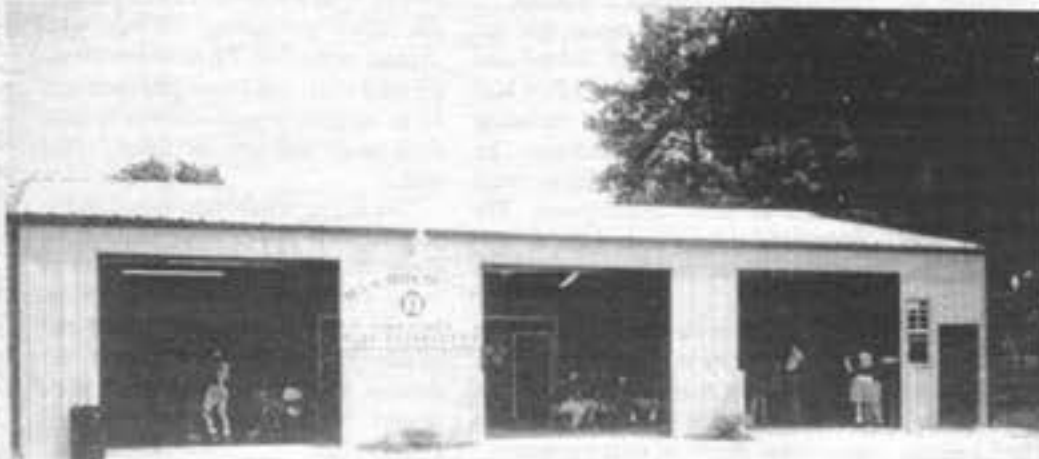
Hammondville Volunteer Fire Department new building
