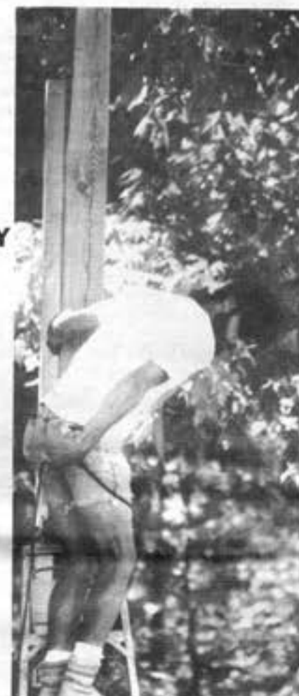
Glen Hansen works on the first slide tower
