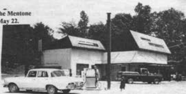
A look at the Mentone Superette from the outside. New gas pumps and a concrete drive way. Business as usual began early Saturday morning. (Photo taken later in the day.) The canopy (not shown) was installed on Wednesday, May 26.
