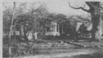
(2) COTTAGE IN VALLEY HEAD. All interior remodeled and freshly painted. Pine Floors and antique doors. New Vinyl siding. 3 bdrm, 1 bath, Butcher Block counters and all appliances. Lots of windows in Living Room and Sunroom. C/H/A. All on 4 acres with Large Shade trees. $93,500.
