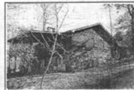
CLOUDLAND - Beautiful two story home overlooking the east fork of Little River sports 3 BR, 1 BA, kitchen, formal dining, great room with stone fireplace, screened porch overlooking river, wet bar and mountain stone fireplace, 2 car garage, shop, and storage area, plus large unfinished attic. 2.5 +/- acre tract, showcased by mountain laurel, rhododendron, and natural beauty of the mountain. Too many amenities to list, and priced at only $129,000. (No G-57)
