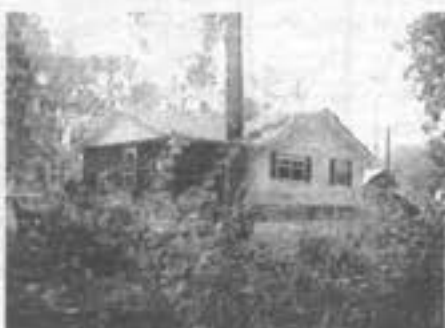
Chattooga Drive - Lake Weiss lake front, neat 2 BR, 1 BA, newly remodeled, vinyl, windows, hardwood, berber, CHA, screened porch, dock, seawall, double lot, private, great area. $150,000.
