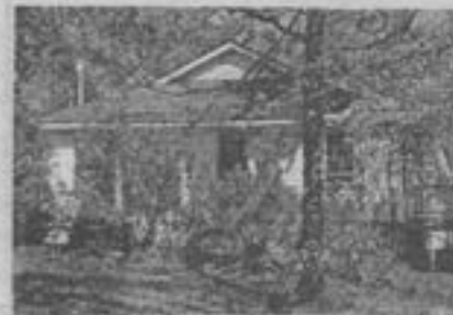
(6) MENTONE FARMHOUSE. with 4.46 acres to Roam. 2 Bdrm 1.5 bath. Country Kitchen, Pine Floors throughout. Deck and outbuildings. Newly Re-wired, plumbed, C/H/A, Vinyl siding and a Root Cellar. $118,500.
