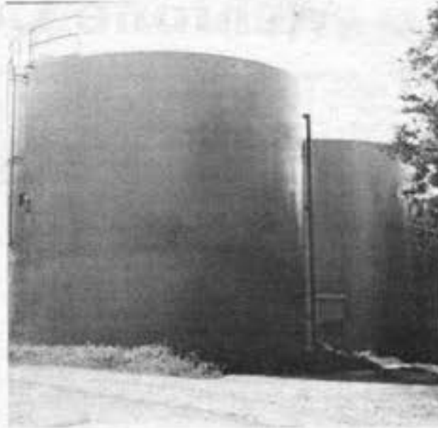
The New Water Tank has been painted and is being tested.
