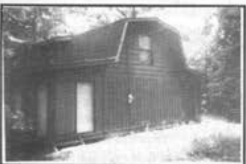
(10) VACATION HOME ON LITTLE RIVER CANYON - Loft bedrooms, 1-1/2 bath, with 7.5 acres and a creek that runs across the property. $68,000. Canyon View Forest (SUB).
