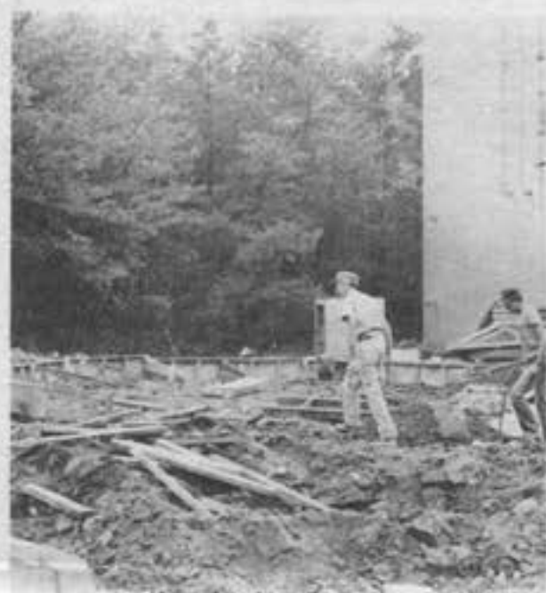
The new water tank is almost completed. Construction had just begun when this photo was taken. There will be a fence around both tanks; the old one is being scraped and painted.
