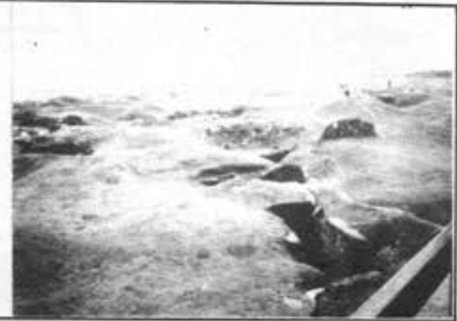
Bunkers left from Normandy Invasion in WWII
