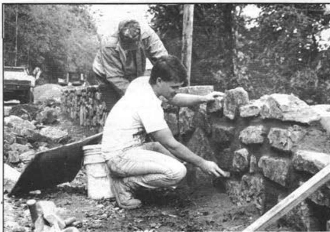
PUTTING UP THE WALL: Pictured working on the rock wall at Mentone are Heath Miller, front, from Fyffe, and Tim Treece, from Huntsville. Both work for Southeastern Landscape. The historic wall along Highway 117 was in need of repair. The Alabama Department of Transportation closed one lane of the highway while the repairs are being made. Traffic has been temporarily diverted to traveling up Tutwelter Gap and traveling down the mountain in the north bound lane of Highway 117.
