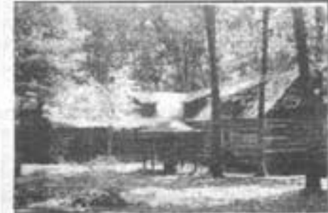
(8) ADIRONDACK STYLE (1800'S) LOG LODGE sitting on 2 private acres in downtown Mentone. Complete with Dog Trot separating the Kitchen with Fireplace and Living Area with Fireplace. Unique 4 Bdrm, 2 Bath. Screened Breezeways, and Porches. Wood Floors, and Tin Roof. Separate Guest Cottage. City Water, along with Hand pump Well. Step back in time with this One-of-a-kind FURNISHED HOME. Reduced to $137,000.
