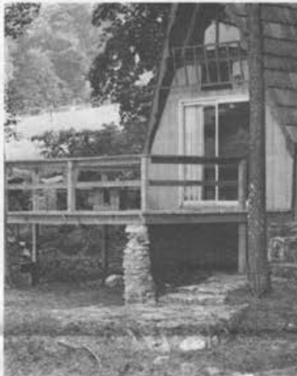
Chalet Number 4 at Cloudmont Ski and Golf Resort sports a new deck. Decks on the other chalets are now being replaced.
