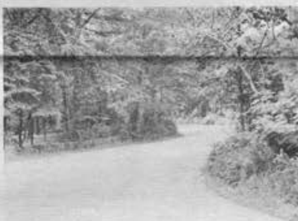
THE GROUNDHOG camera caught the above scene from the newly resurfaced DeSoto Parkway, to which has been applied layers of tar and gravel, topped off by a second layer of tar and finer gravel. Many complaints had been registered concerning the rough surface and potholes along the Parkway.
