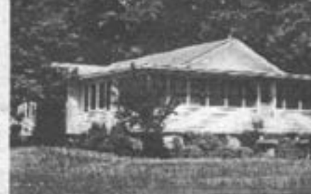
(10) TRULY THE MENTONE LOOK. Great commercial building on Hwy 117. Open rooms with pine floors and Tung and Groove Walls. Kitchen, bath. Built-in Shelves and Counters. All new wiring and plumbing. Glassed Porch. Open your own business in Downtown. $123,000.
