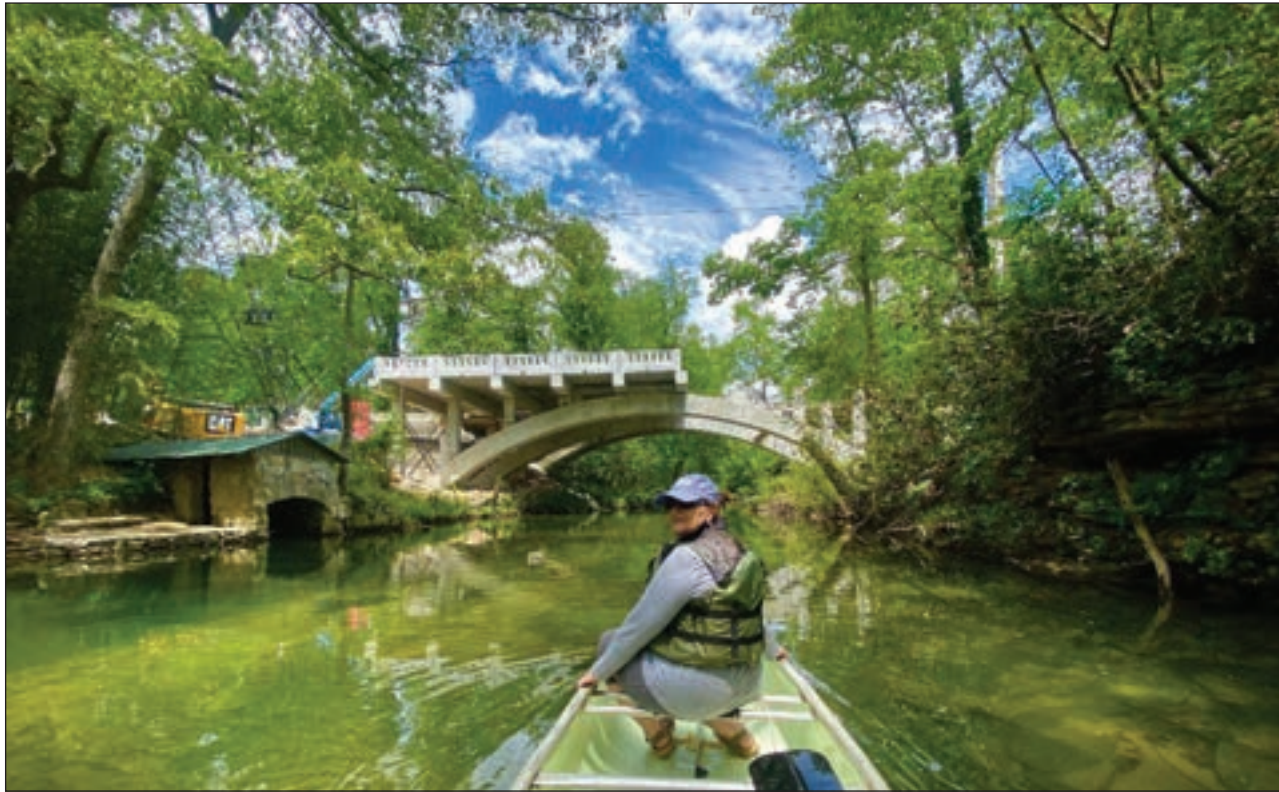
My wife, Beverly, and I paddled our canoe up the West Fork of Little River to the new Highway 117 bridge (currently under construction). It was a beautiful day for a lazy float amongst the rhododendron and mountain laurel. —Photo by David Haynes, May 14, 2020
