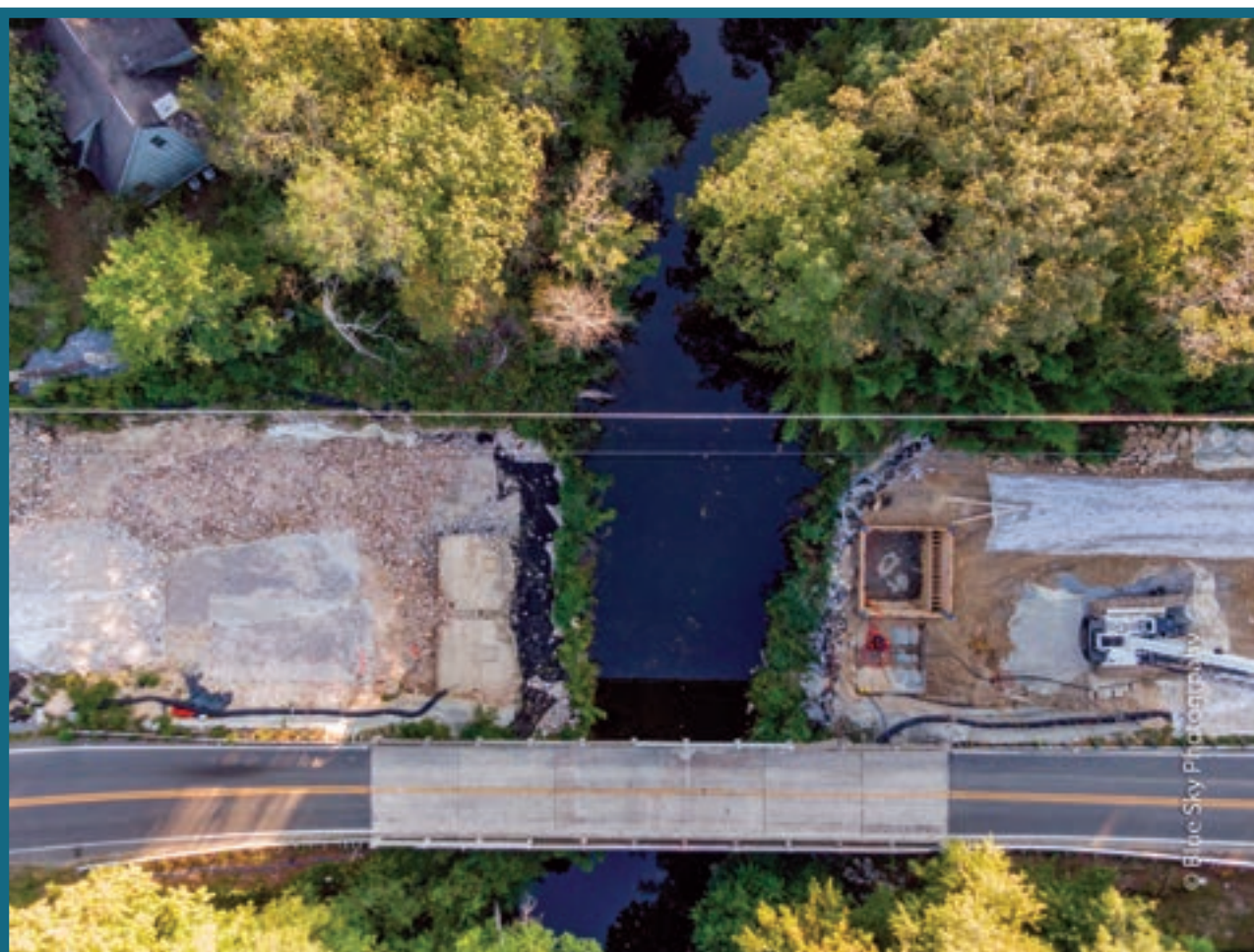
A drone photo taken by Charlie Stone of Blue Sky Photography on September 15, 2019, shows a bird's-eye view of the bridge construction on AL Highway 117 over the west fork of Little River. The bridge is slated to be complete later this fall.
