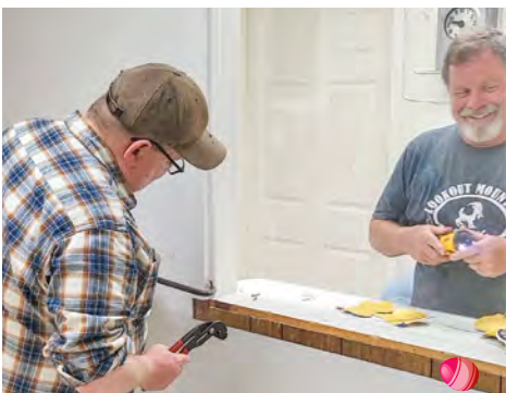
LRAC board members Stephen Smith and Mikel Yeakle working on the Little River Art Gallery one year ago.
