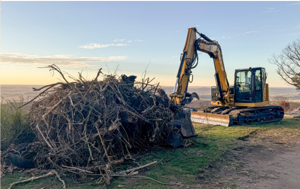
Crews are removing underbrush from along the bluff below Brow Park. Next year, additional phases will bring a walking path, observation deck, and hiking trails off the bluff to this popular park. The work depends on grant awards.
